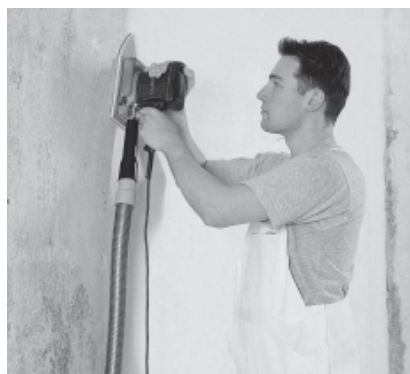
Vacuuming dust when working with electrical tools controlled by power-up of the vacuum when the electrical tool starts. (order number 58 405 1)
